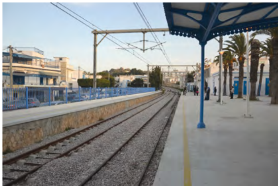
Station La Marsa, terminus du TGM © CODATU
