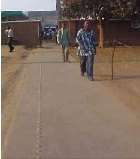
Figure 5: Upgraded footway with tactile path, Blantyre
