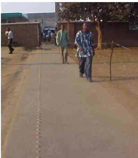
Figure 5: Upgraded footway with tactile path, Blantyre
